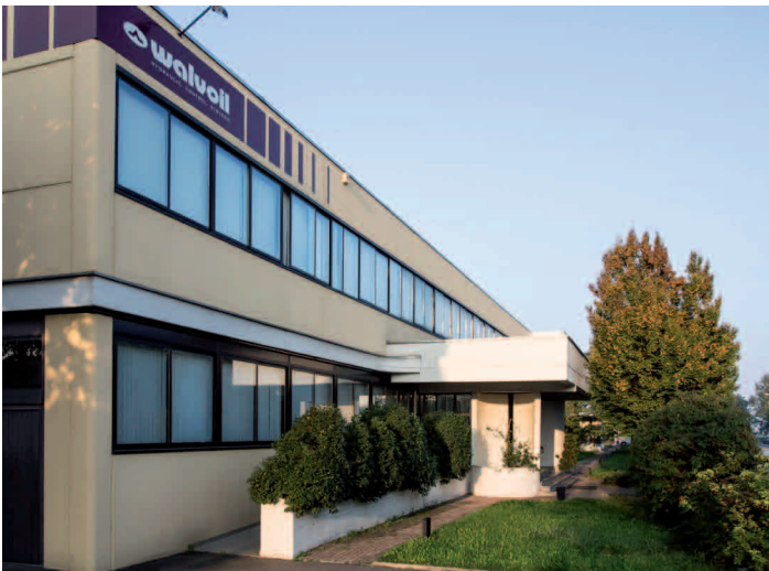
W2 usinagem W2 mechanical machining
